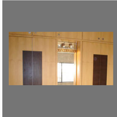
Interior Wood Work
